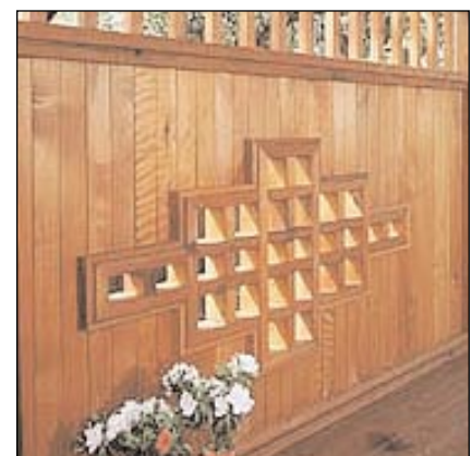
Privacy screen surrounding a built-in spa features an intricate cutout framed with a series of 2x4 boxes. Gentle breezes and filtered light keep the space from feeling dark and confined.
