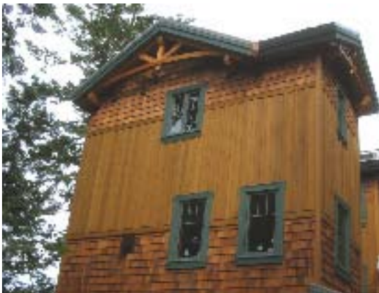
Red Cedar sidewall shingle siding and channel siding Pictures by Cloud Bannick Builder: Ravenhill Construction
