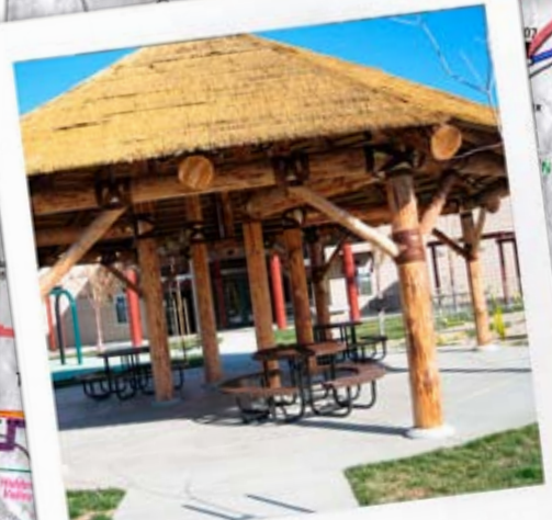
Douglas Fir peeled logs Tachi-Yokut Tribe Center Lemoore, CA
