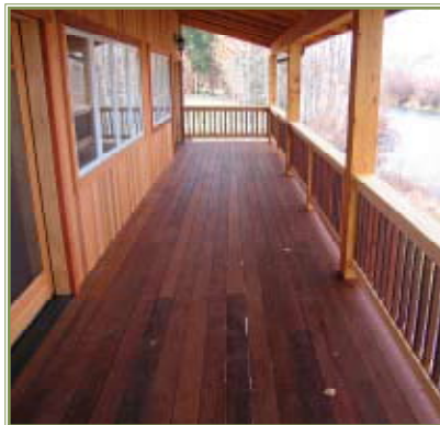
Opposite page: Before and after pictures of what Bear Creek Lumber can do for your remodel. Below: Ipe hardwood decking is beautiful and is one of the hardest decking materials available. It is also fire and rot resistant, making it an excellent investment. James finished the Ipe with a couple coats of Seafin. Right: Douglas Fir rafters.
