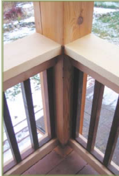
Left: Douglas Fir Posts and soffit. Center: A Hemlock rail cap, with Ipe railing connects to a Western red cedar Post. Top Right: Port Orford cedar Interior paneling. Middle: Generous porches that wrap around with Ipe decking.
