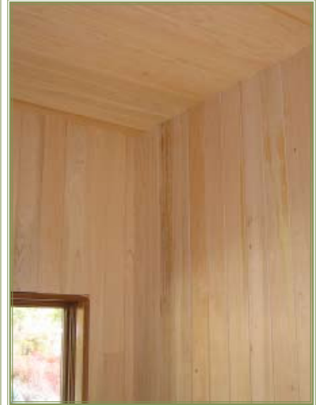
Left: Douglas Fir Posts and soffit. Center: A Hemlock rail cap, with Ipe railing connects to a Western red cedar Post. Top Right: Port Orford cedar Interior paneling. Middle: Generous porches that wrap around with Ipe decking.
