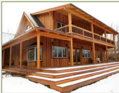
Opposite page: Before and after pictures of what Bear Creek Lumber can do for your remodel. Below: Ipe hardwood decking is beautiful and is one of the hardest decking materials available. It is also fire and rot resistant, making it an excellent investment. James finished the Ipe with a couple coats of Seafin. Right: Douglas Fir rafters.
