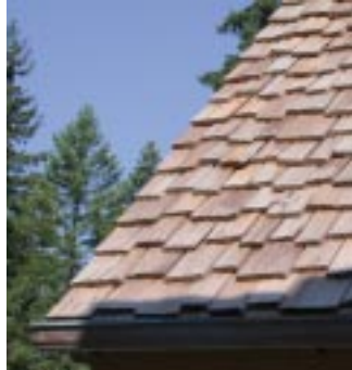
Right: Close up view of the 24" #1 Heavy fire-treated cedar shakes. These have weathered for about one year.
