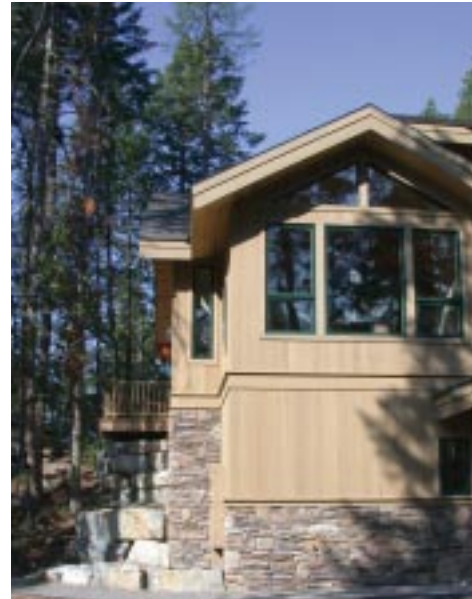
Above: The Dow residence. Siding was 1 X 6 Western Red Cedar A&Btr. clear T&G flush joint with a resawn face. BCL also provided pre-staining.
