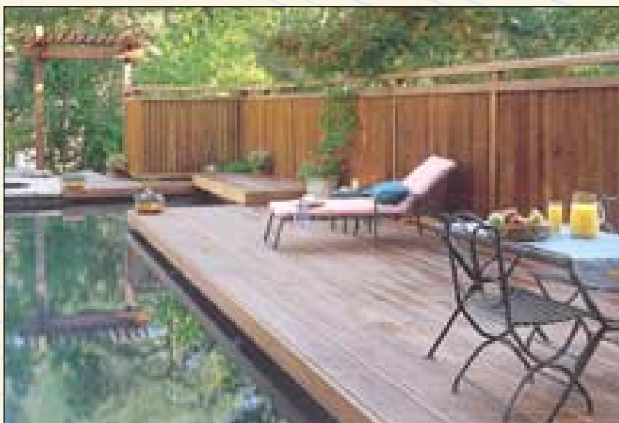
Louvered poolside privacy screen. Graceful, seven-foot-high redwood fence screens a pool from surrounding houses. The pool also features a multi-level redwood deck that appears to float at its edges. Fence boards were louvered to allow views of the landscape while creating a property line barrier.
