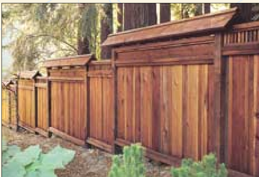
Gabled hillside fence. A series of Construction Heart/Deck Heart panel modules are stepped along a sloping site. Intriguing fence top design consists of alternating inserts of uprights and gabled roofs.
