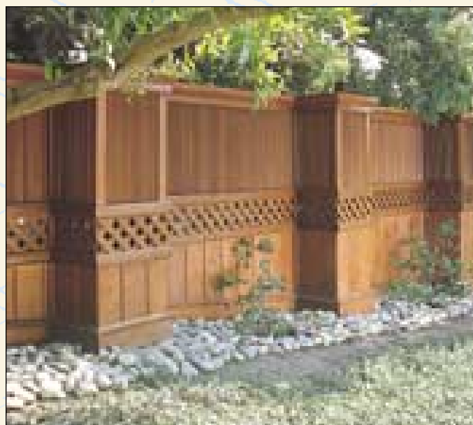
Handsome columned fence. Intricate design consists of tongue and groove boards topped by a strip of redwood-ribbed lattice and then by louvers which are set at a 45° angle.
