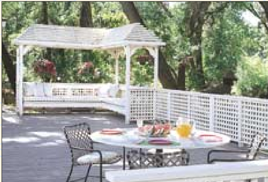
Corner bench deck shelter. L-shaped bench transforms a bare corner of a deck. The 9x9 structure has a hip roof that creates a shady retreat. Classic redwood lattice panels form the back of the bench, echoing adjacent deck railings.
